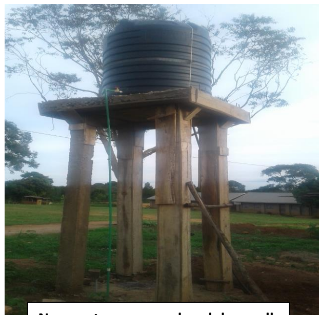
New water source – hand dug well with solar pump, water storage tank and tap!
